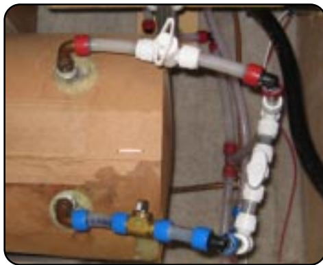
Water heater by-pass valves
