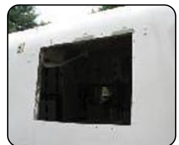
Window opening ready for window installation.
