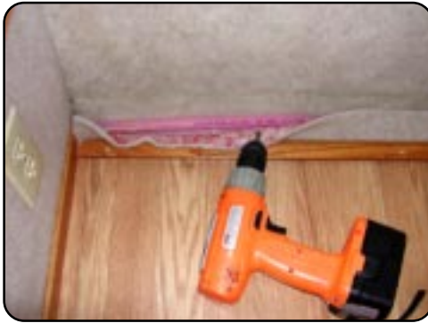
Back area and plumbing cover up.
