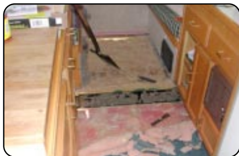
View of carpet tearout.
