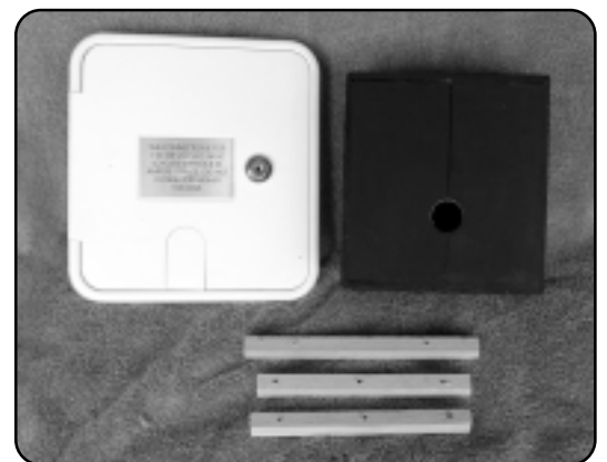
Photo 2 - The new power cord housing with a locking door. The black wooden box on right fits into the back of the plastic housing and is secured with short screws. The part with the power cord hole is in two pieces. After the housing is installed with one side in place, the power cord is pass through and the second side secured in place. The three small wooden strips are sized and fitted to go inside the trailer to receive the screws used to mount the housing to the Scamp's fiberglass skin.
