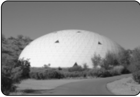
Two massive spherical domes like this one served as “lungs” for Biosphere 2 allowing the internal spaces to “breathe.”
