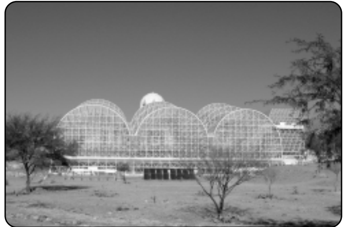
This view of Biosphere 2 illustrates the massive amounts of glass necessary to enclose the structure.
