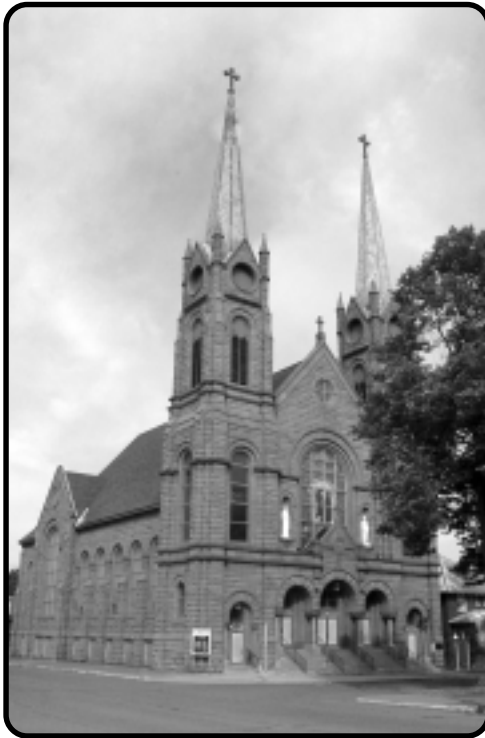
This large church is typical of many buildings in downtown Calumet - some more than a hundred years old. It is composed of Jacobsville Sandstone, a popular building material used during the copper mining era.
