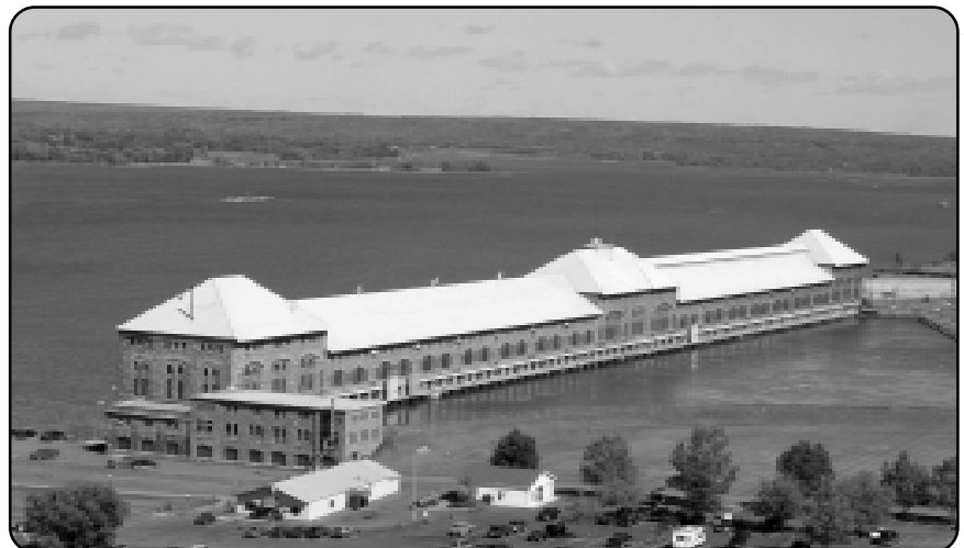
Edison Power Plant – This hydroelectric generating facility, located below Soo Locks, uses a difference in elevation between Lake Superior and Lake Huron. It is made of Jacobsville Sandstone, removed from the canal that feeds the plant.
