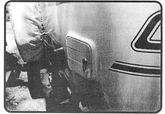
There may be as much as 1/8 inch of plumbers putty and caulk to fill the gap between the round trailer side and the straight door frame.
