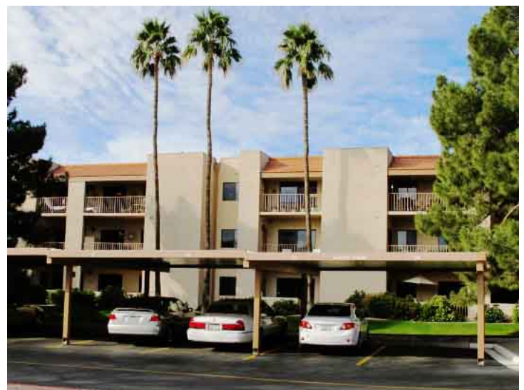
Royal Oaks is a 3 story facility
